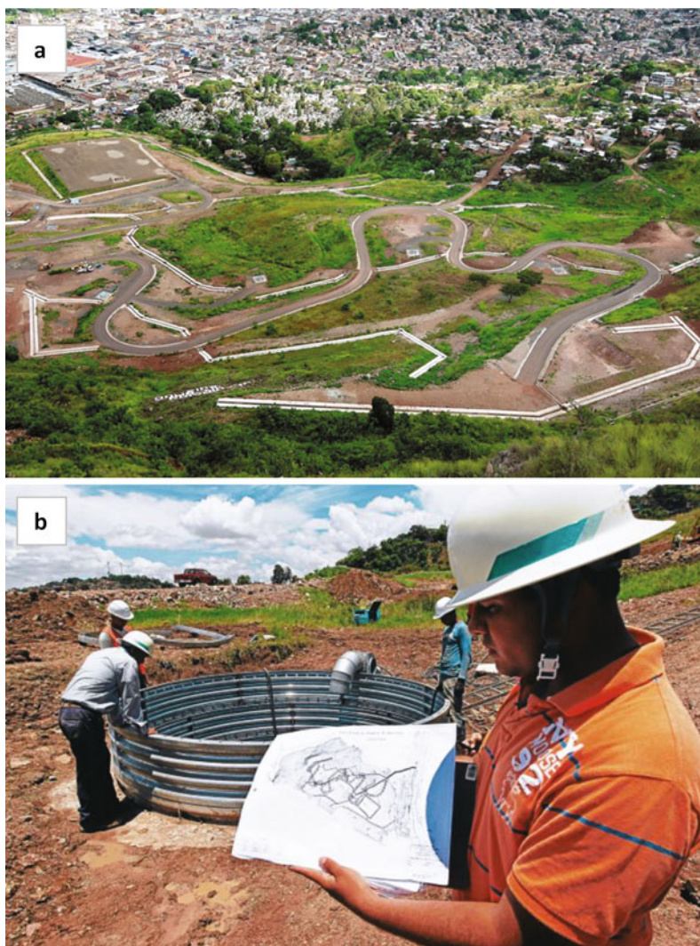
Fig. 9.7 Countermeasures carried out by JICA to reduce the landslide risk in El Berrinche Hill. a Channels that transport surface water are shown. b One of the drainage wells with intake pipes at different depths to collect groundwater is shown. Both figures were taken from El Heraldo newspaper and were published on April 7, 2014
