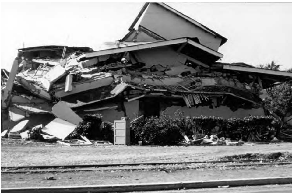
Figure 89 Nicaragua earthquakes December 1972, Managua, collapsed the three-story, reinforced concrete Customs House office building.
