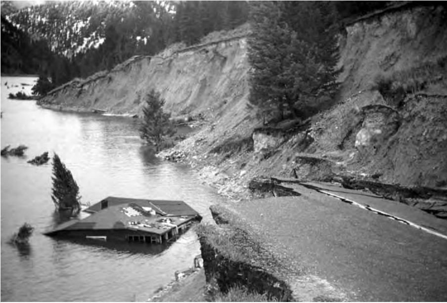
Figure 74 Hebgen Lake, Montana, earthquake, August 1959. Slump of former State Highway 287 into Hebgen Lake. The main residence of Hilgard Lodge is almost wholly submerged in the lake. View is northwestward. August 1979.
