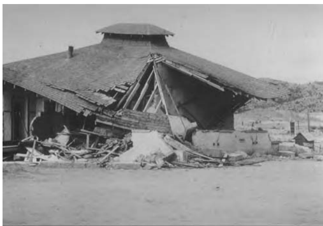
Figure 66 Collapsed school in Kern County, California, earthquake, 1952. The Cummings Valley School completely collapsed. The school building was reportedly constructed in 1910 of concrete walls and a wood roof. The building was a total loss.
