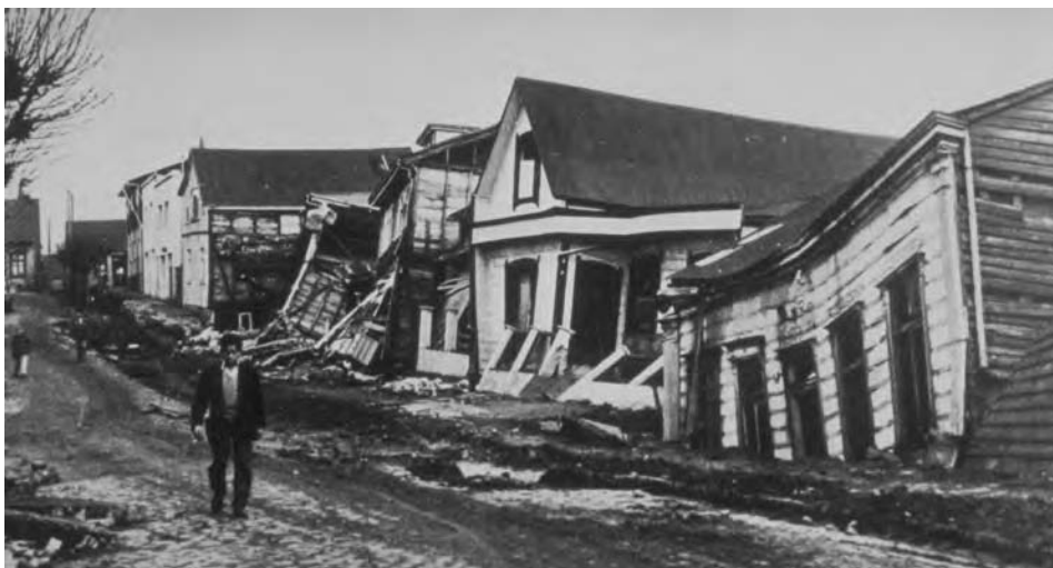
Figure 76 Waterfront street in Quellon (located on the eastern shore of Isla Chiloe). The half-demolished building was the city hall. This part of Isla Chiloe sank about 6.5 feet. Some houses near the sea had to be evacuated; water reached the main street of the town.
