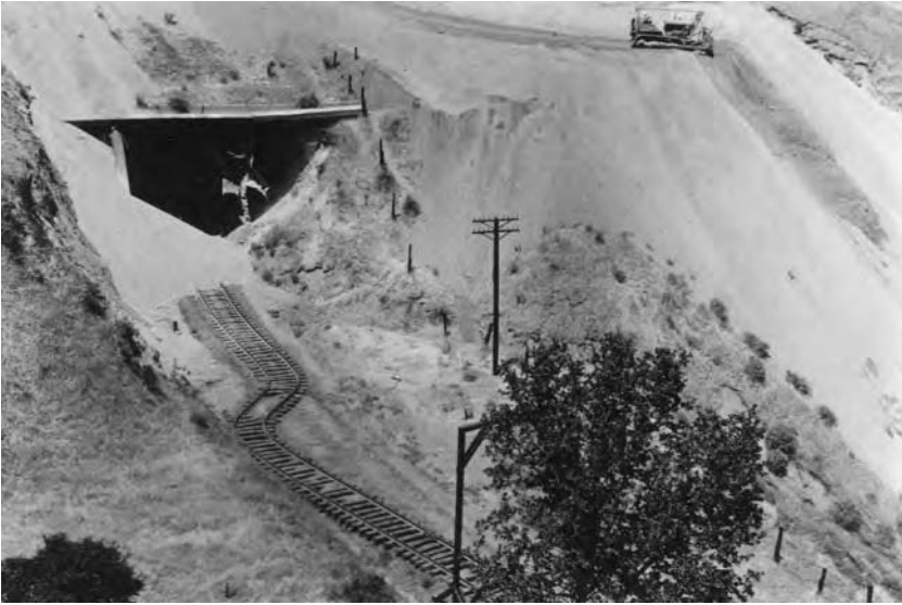
Figure 67 Earthquake damage along the Southern Pacific Railroad near Bealville. Sharp bend in the tracks south of Tunnel 3 strikingly demonstrates that the ground had been shortened in this area. A landslide blocks the east portion of the tunnel.
