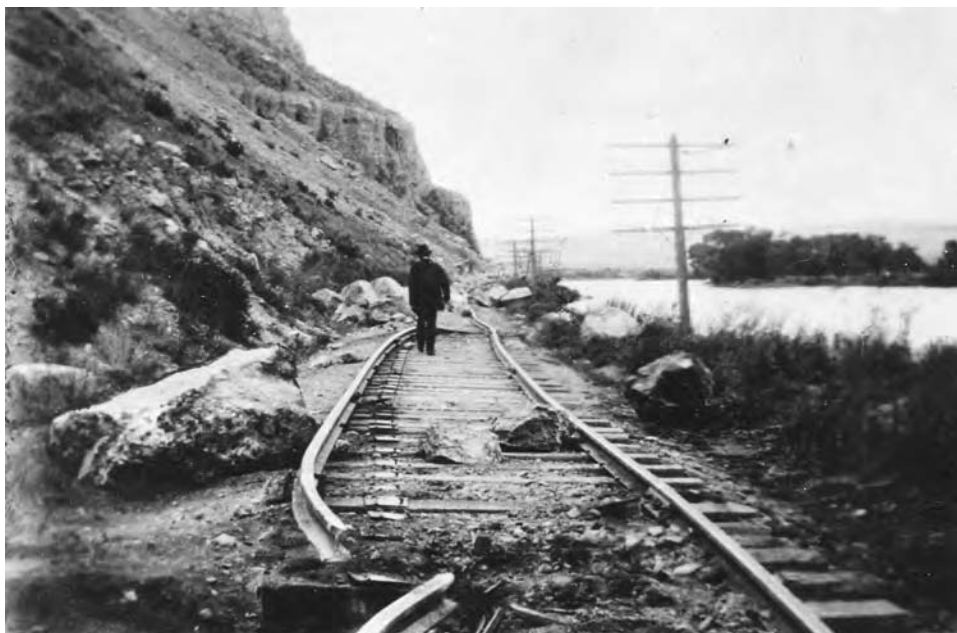
Figure 49 Montana earthquake of June 27, 1925. Broken railroad track near Lombard.
