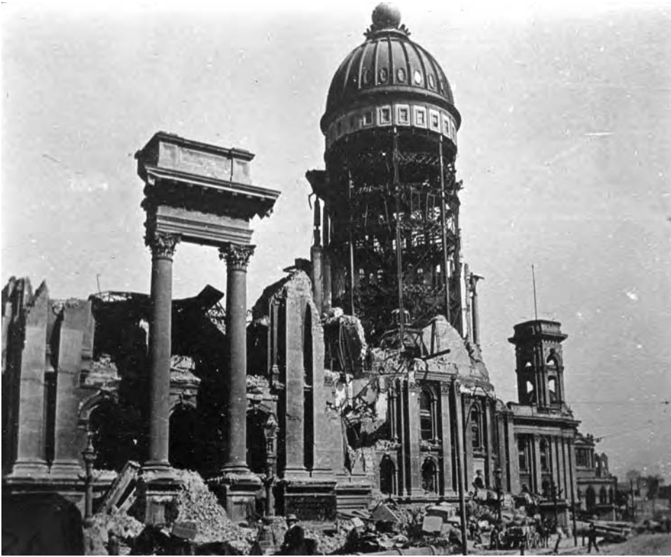
Figure 37 San Francisco, California, earthquake, April 18, 1906. View showing damage the San Francisco City Hall resulting from the San Francisco earthquake and fire of 1906.
