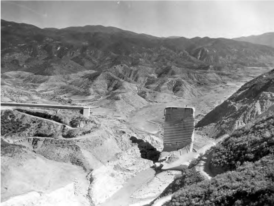
Figure 52 St. Francis Dam flood, March 12–13, 1928, Los Angeles County, California. Taken from the same location, showing the remains of the dam and reservoir floor. The dam failed at 1:58 P.M. Monday, March 12, 1928, according to the water storage recorder on the dam. Twenty minutes prior to that time, the water was slowly dropping in the reservoir indicating that leakage was increasing. The flood destroyed the power house about one mile below the dam at 12:04 A.M. March 13, 1928. The left (west) abutment of the dam was entirely swept away.
