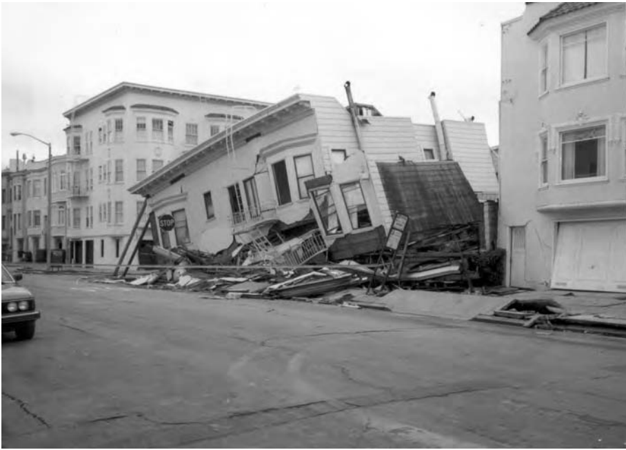
Figure 108 Loma Prieta, California, earthquake, October 17, 1989. Structures damaged in the Marina District of San Francisco. The first story of this three-story building was damaged because of liquefaction; the second story collapsed. What is seen is the third story.
