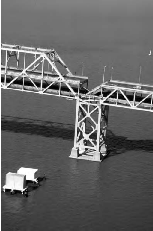
Figure 107 Loma Prieta, California, earthquake, October 17, 1989. Road-bed collapse near the interface of the cantilever and truss sections of the San Francisco–Oakland Bay Bridge.
