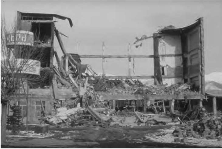
Figure 105 This is the five-story communications building in Spitak. It is a pre-cast, concrete-frame composite structure. Many of these structures collapsed contributing to the high death toll.
