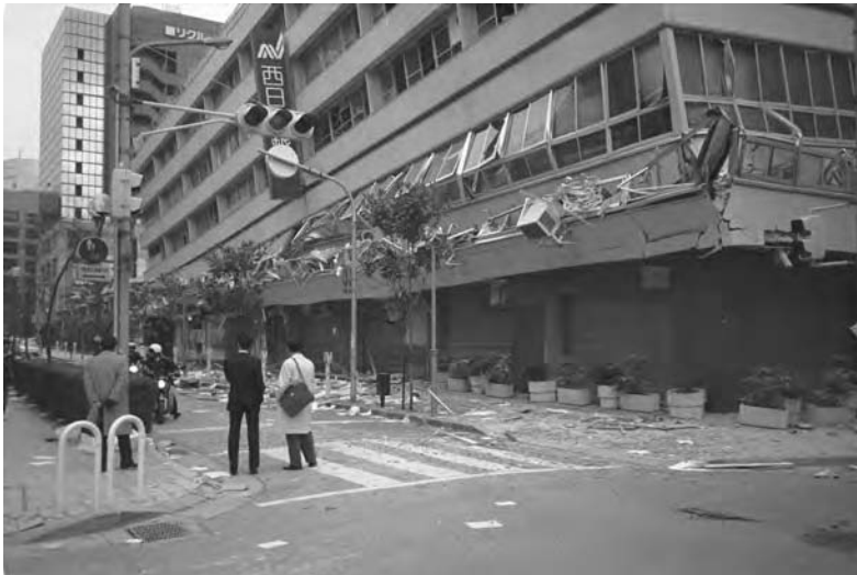
Figure 118 The first and second stories of a metal frame office building collapsed. This photo demonstrates the lateral force of the quake and the structural damage caused by the sine wave effect of the force. Note the unbroken windows.
