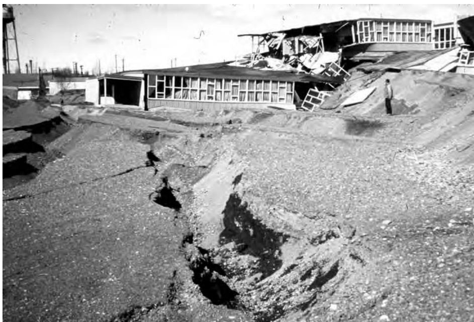
Figure 80 Alaska earthquake, March 27, 1964. Government Hill Elementary School in Anchorage which was destroyed by the Government Hill landslide.
