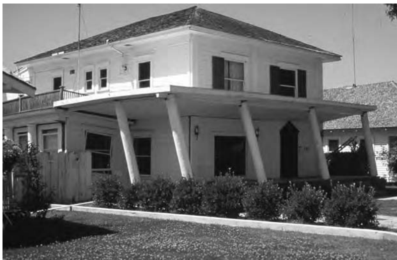
Figure 101 Coalinga, California, earthquake, May 2, 1983. House displaced from its foundation, as shown by movement of its columns. The house was in the restricted area of heavily damaged downtown Coalinga. May 7, 1983.
