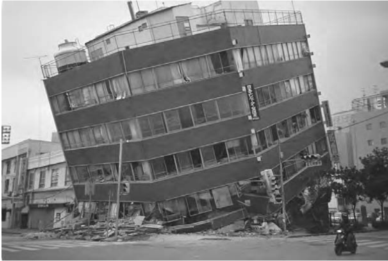
Figure 117 An office building with a partially destroyed first floor. The majority of partial or complete collapses were in the older, reinforced concrete buildings built before 1975.
