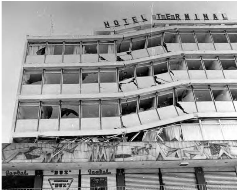
Figure 93 Guatemala earthquake 1976. Collapse of the Hotel Terminal in Guatemala City, caused by the failure of reinforced concrete columns in its third story. 1976.
