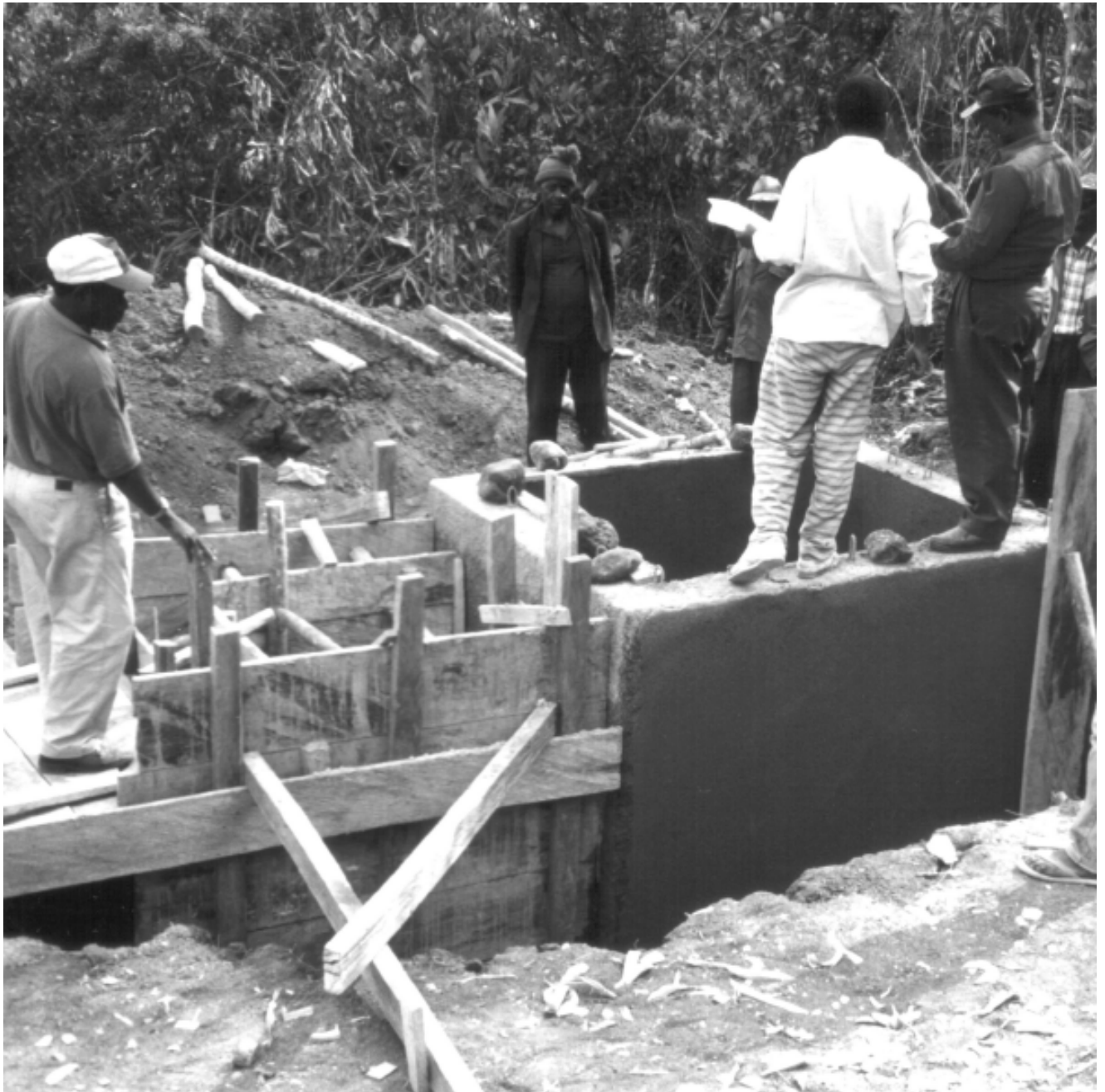
Construction of a spring chamber
